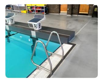
different cleaning and slip resistance priorities. By using epoxy systems, the specified coating doesn't need to change in different areas, just the amount of aggregate broadcast into the floor's resin matrix.
