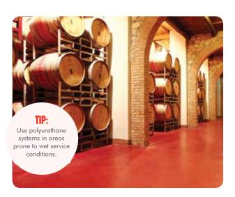
Different textures can be used and the floor can be broadcast with aggregates to improve its anti-slip properties. Coarsely textured surfaces are more difficult to clean so if you require both an anti-slip and easily cleaned surface you must consider the priorities of your venue before confirming a floor choice.
