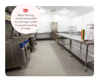
In wet service environments, it is essential that flooring is laid to falls leading to an efficient drainage system in order to prevent the pooling of water and heighten the risk of slips.
