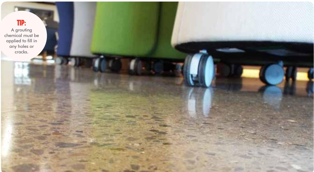
Polished concrete floors are susceptible to moisture and need to be properly sealed on both the top and the bottom. If liquid does manage to infiltrate the pores of the concrete then it could cause mould and mildew to grow, and if the liquid freezes it could lead to serious cracking in the slab.
