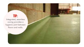
smooth and level to allow for effective cleaning but also highly durable to withstand the intensive maintenance.
