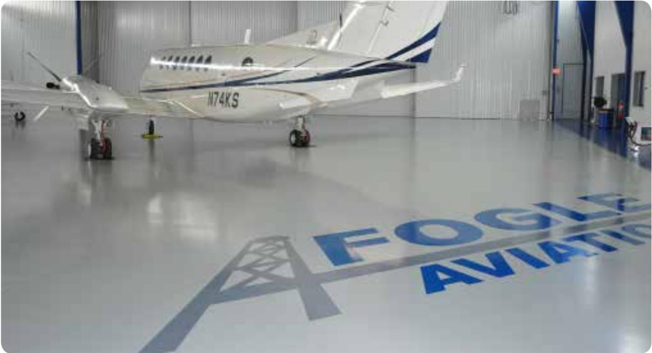
Anti-slip aggregates can be included within the resin make up of an epoxy system to provide extra grip underfoot. The anti-slip profile of the floor can even be tailored to meet the varying requirements of different areas of the hangar complex.
